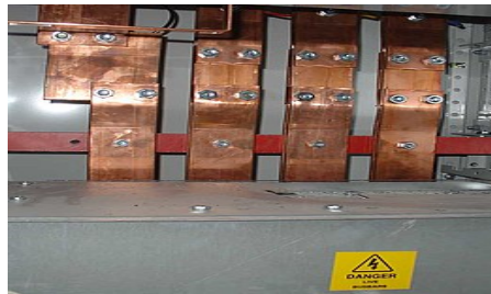
Figure 2.3 Bus bar
