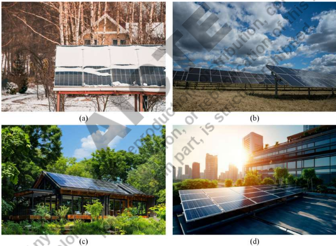
Fig. 12.12 Partial shading scenarios due to: (a) snow, (b) passing clouds, (c) trees, and (d) neighbouring buildings
